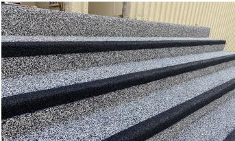
Rubaroc bonds directly to any solid substrate material including concrete, asphalt, epoxy, stone, brick, wood, and more. Surface blemishes are easily filled and eliminated. There is simply no other surface like it!
